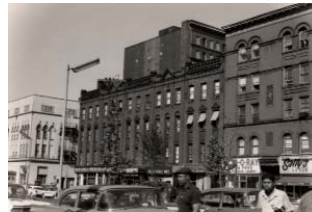
Photograph of 125th St. and Lenox Ave. taken by Margot Gayle in 1961
