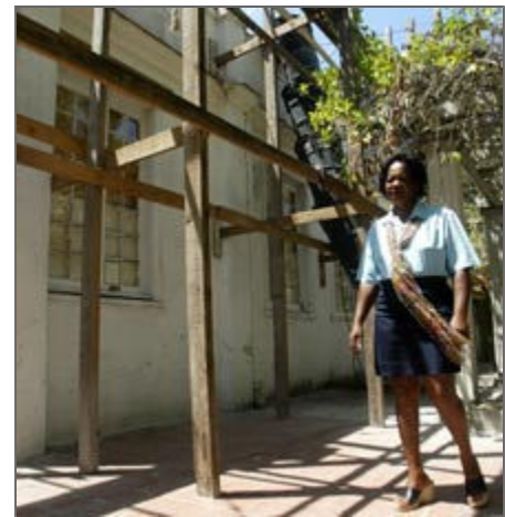
Hemingway's crumbling Cuban home must be bolstered by wood scaffolding. (AP file photo)
