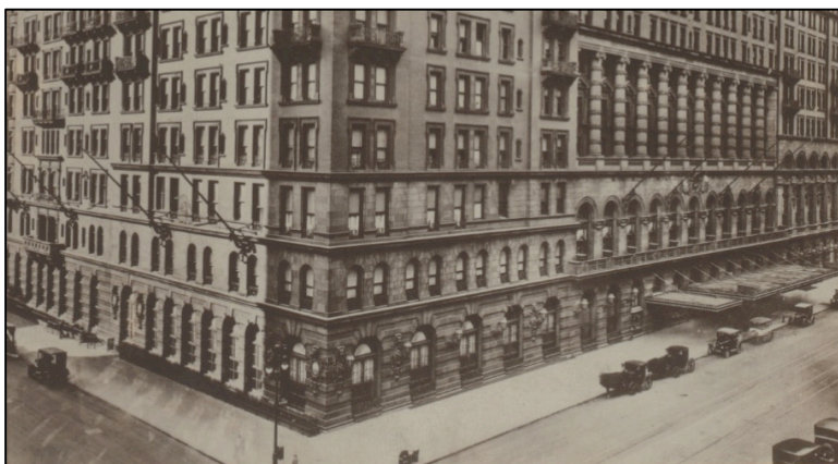
Figure 19. This image shows the base of the Waldorf-Astoria Hotel ca. 1920. The plantings are gone, and the porte-cochere has been removed and replaced with an overhanging canopy, typical of the changes that were made after sidewalk encroachments were removed.
