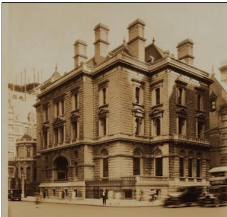
Figure 36. The Huntington mansion lost its entrance staircase and courtyards when the encroachments were removed by street widening, and the bay window facing 57th Street also had to be removed.
