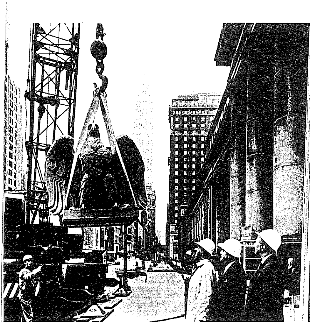
The demolition of Pennsylvania Station.
