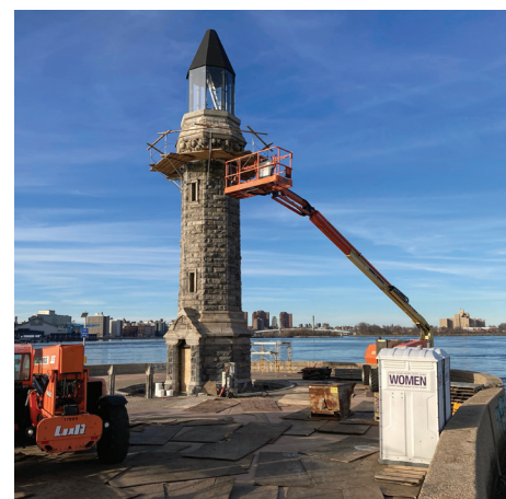
Ongoing 2022 replacement of lantern and restoration of the Roosevelt Island Lighthouse designed by James Renwick, Jr. in 1872. | Courtesy of John C. Harris
