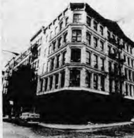
With its cast-iron facade, its columned windows and triangular pediment, 109 Prince St. is a classic example of the SoHo architecture. Phot. Philip J. Frank Lorraine
