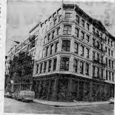
With its cast-iron facade, its columned windows and triangular pediment, 169 Prince St. is a classic example of SoHo architecture.
