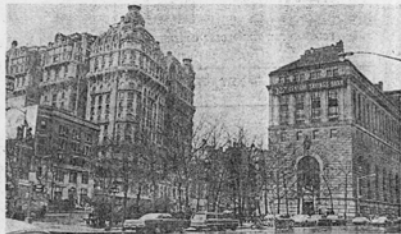
The Ansonia Hotel, at Broadway and 73d St. (l) was saved after a long and heated campaign. But the Central Savings Bank, its distinguished neighbor across the street, was denied landmark status.
