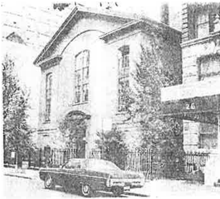
Post Photo by Terence McCarlen The Brotherhood Synagogue, formerly the Friends Meeting House, at the southeast corner of Gramercy Park.
